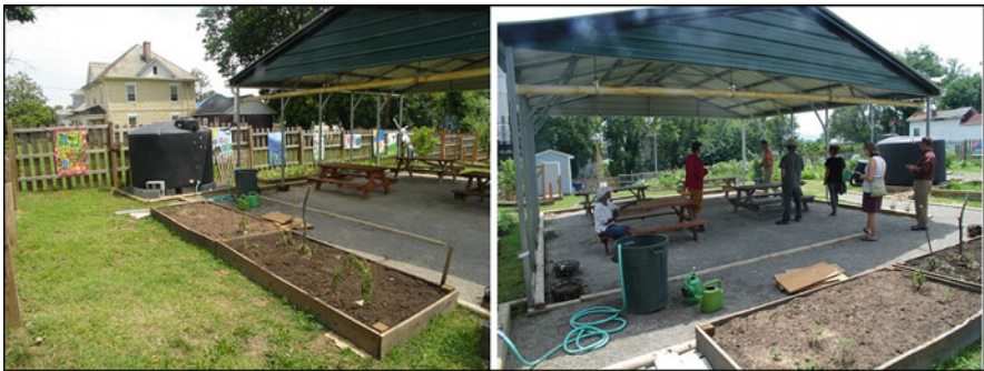
Fig. 9 Rainwater harvesting systems at Hurt Park Community Garden, photo on the left shows a 1500 gal (5.7 m 3 ) barrel to the left of the pavilion; photo on the right shows a second barrel to the right of the pavilion (Photos: Third author 2013)
