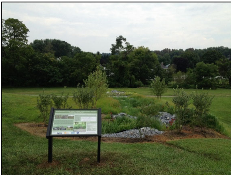
Fig. 17 Regenerative stormwater conveyance (Source: Center for Watershed Protection)
