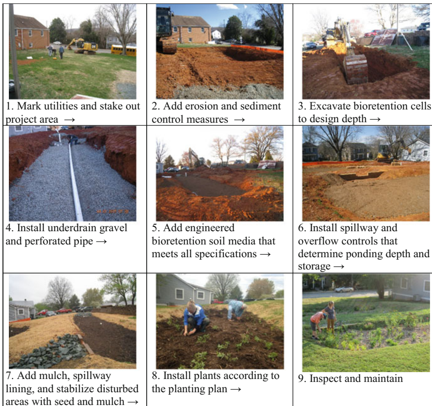
Fig. 21 Typical installation sequence for bioretention (Source: first author)
