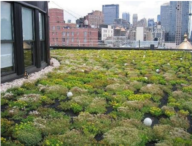
Fig. 19 Vegetated roof ( Source: West Virginia (USA) Department of Environmental Protection )
