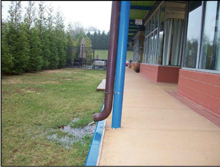
Fig. 11 Simple impervious surface disconnection ( Source: first author )
