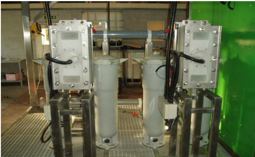
Fig. 2.39 Showing two, multiplate diamond electrochemical reactors for industrial scale water treatment
