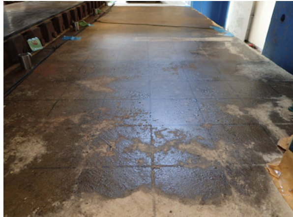
Fig. 4 After repair agent execution
