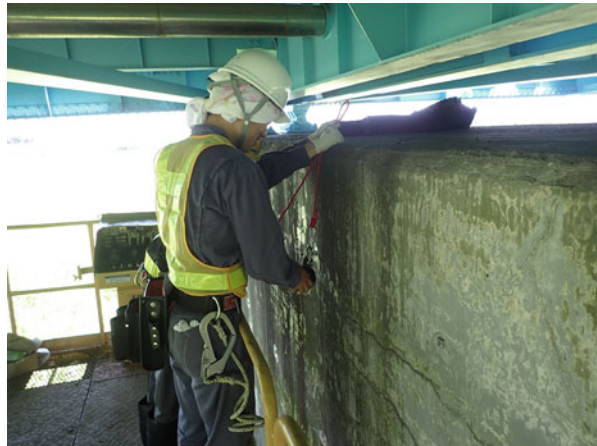
Fig. 2 Elastic wave excitation with impacting a ball on concrete surface (right)
