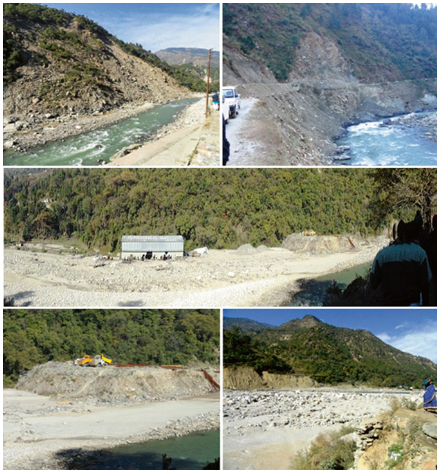
Fig. 12.3 The number of massive landslides has been activated on both sides of the valley, and the powerhouse site of (L&T) is completely covered by debris (Source: Author)
