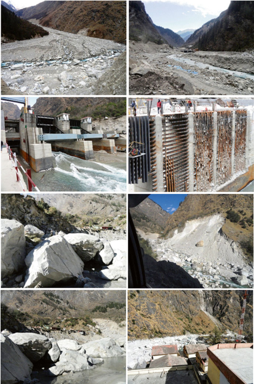
Fig. 12.8 Photograph showing the fury of nature in Alaknanda valley (Source: Author)
