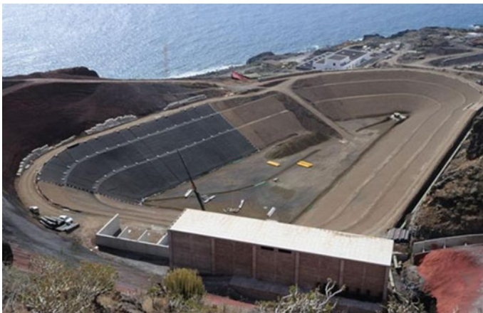
Fig. 10 Lower deposit in construction (Gorona del Viento, with permission)
