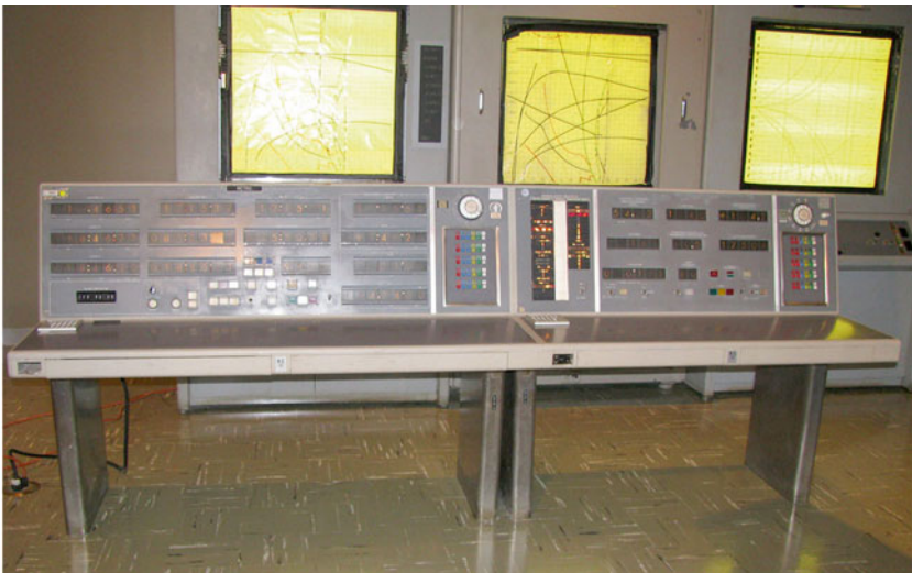
Fig. 14.7 The restored Retrofire Officer and Flight Dynamics Officer consoles and plot boards. (Photo courtesy of NASA)
