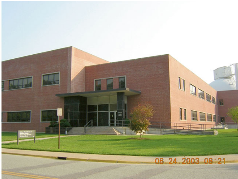
Fig. 7.1 Langley's Unitary Flow Wind Tunnel, Building 1251. (Photo Courtesy of the NASA Langley Research Center)
