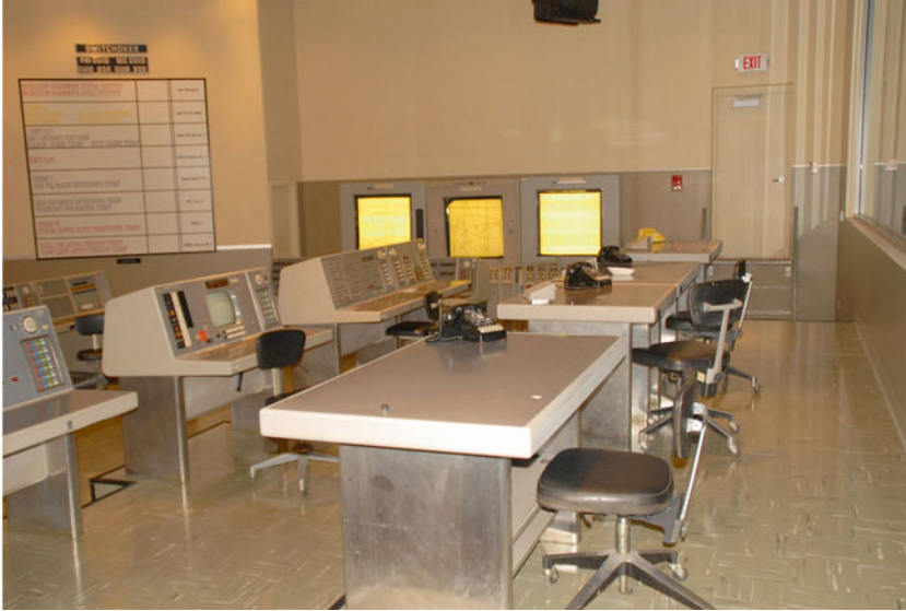
Fig. 14.6 The restored upper row of consoles for the Navy Recovery Task Force Commander, Public Affairs Officer, Operations Director, and Air Force Network Commander. (Photo courtesy of NASA)
