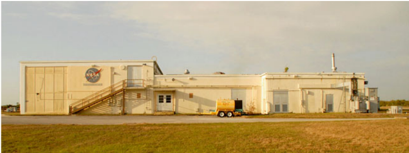
Fig. 14.8 The MCC in 2010 prior to demolition. (Photo courtesy of NASA/Jack Pfaller)
