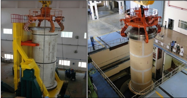
Fig. 22 Segment being lowered into casting pit
