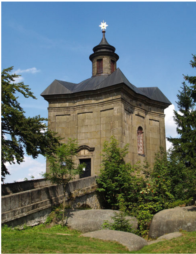
Fig. 17.14 Baroque chapel “Hvězda” (Star) in the central part of Broumov cliffs (Photo J. Vítek)
