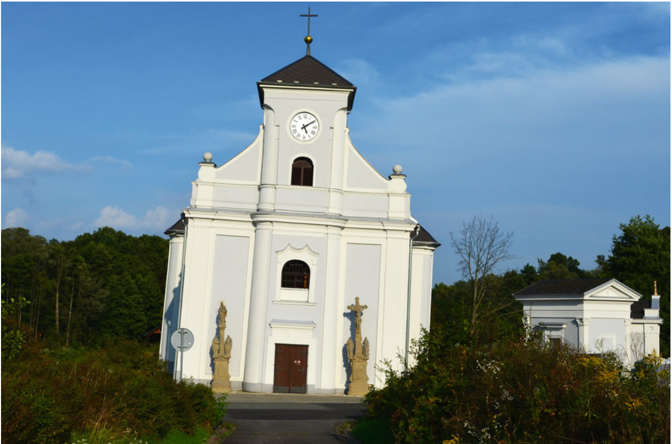
Fig. 25.9 Contemporary view of the Church of St. Peter of Alcantara in Karviná-Doly mining area. The church subsided by 36 m. (Photo M. Mulkova)
