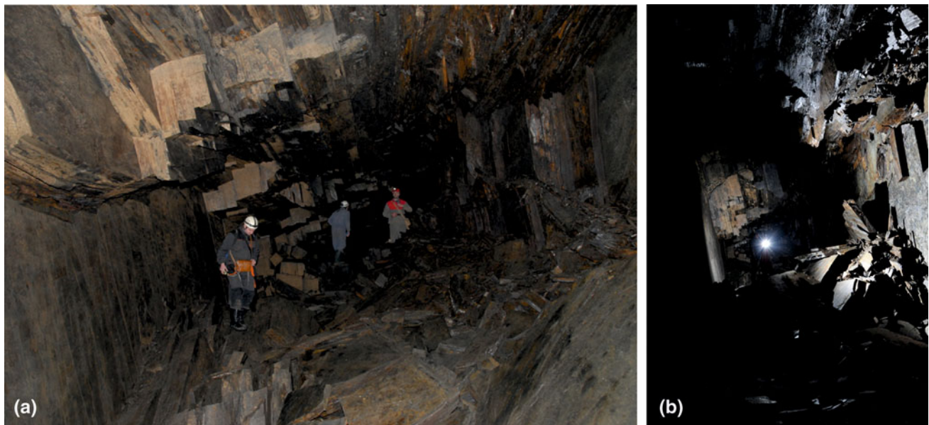
Fig. 24.9 Collapsed rocks within the old mine near the village of Černná ve Slezsku: a the passage is shifted upwards due to collapses of slate plates; b collapsed walls and ceilings in the same mine. (Photo J. Wagner)
