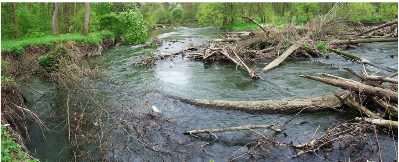
Fig. 23.7 An example of large woody debris accumulation in the dominant channel of the Morava River originating from the erosion of floodplain covered by forest (Photo L. Krejčí)
