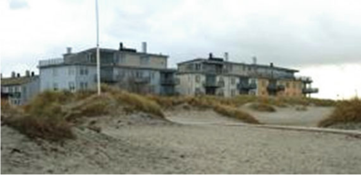
Fig. 9 The Lomma Eternit area today. Photo: Anders Högberg
