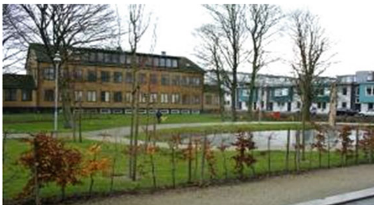
Fig. 8 The office building for Skandinavisk Eternit company. Photo: Anders Högberg
