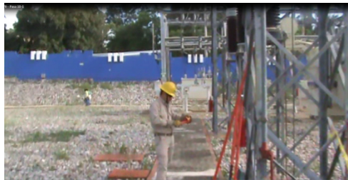
Fig. 2. Bypassing an interrupter. This works is previous to electrical tests performance.
