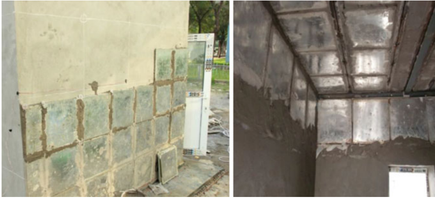
Fig. 9 Demonstration of PCM panels installed for the PCMOW and PCMIW (Kong [36])
