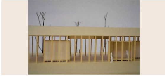
Fig. 57.21 The façade is structured by a row of columns. The inner core is flexible; technical installations are at floor level and in wall panels so that each lab module connects and disconnects as needed
