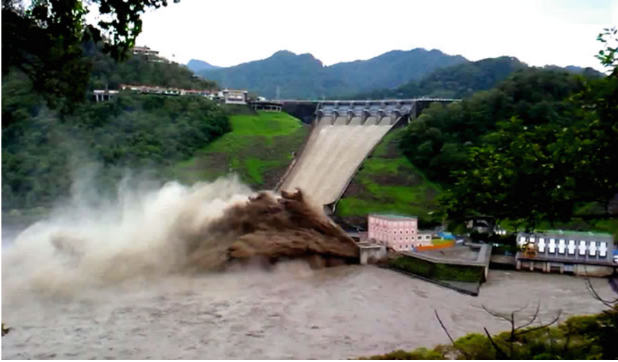
Fig. 10.32 Photo showing muddy water sluiced out from the sluice tunnel as the density current reached the dam
