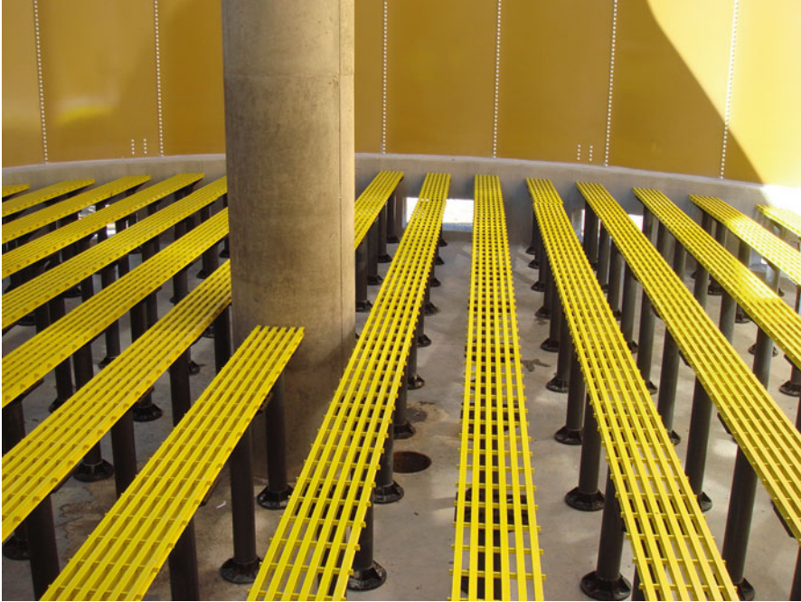
Fig. 6.5 Underdrain system, consisting of plastic stanchions and FRP gratings (Courtesy of Brentwood Industries, Inc.)
