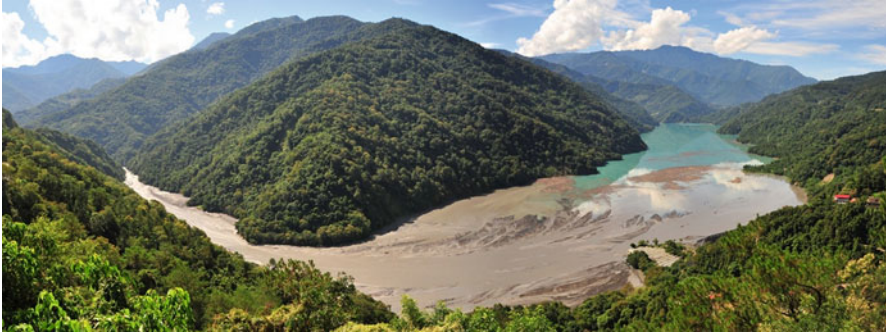
Fig. 10.2 Photo showing large amount of sediments transports to the Wu-She reservoir at hyperpycnal concentrations during Typhoon Morakot in 2009 (Photo taken by Mr. Ke Wun-Tao, Courtesy of Prof. H Capart, Morphohydraulics Research Group, National Taiwan University, Taiwan)
