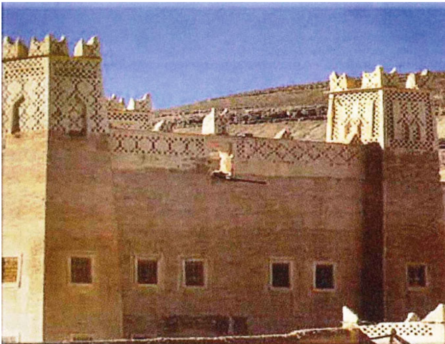
Fig. 22.5 Traditional adobe building in High Atlas
