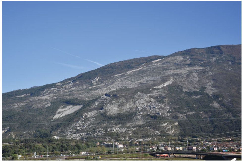
Fig. 9.5 Lavini di Marco landslide. The stratum surfaces along which sliding occurred are clearly visible. The landslide body is recognizable in the slope lower part ( photo G. Carton )
