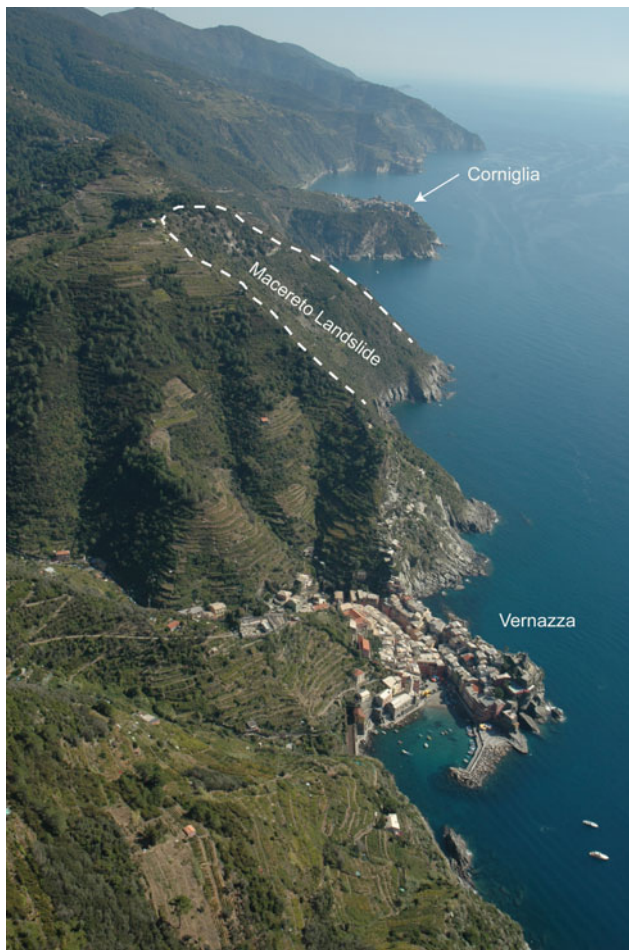
Fig. 20.3 Panoramic view of the Cinque Terre from west: in the foreground the village of Vernazza surrounded by very steep and cultivated terraced slopes; in the background the ancient Macereto landslide and the Corniglia village located on a former marine terrace (photo Cinque Terre National Park Archive)
