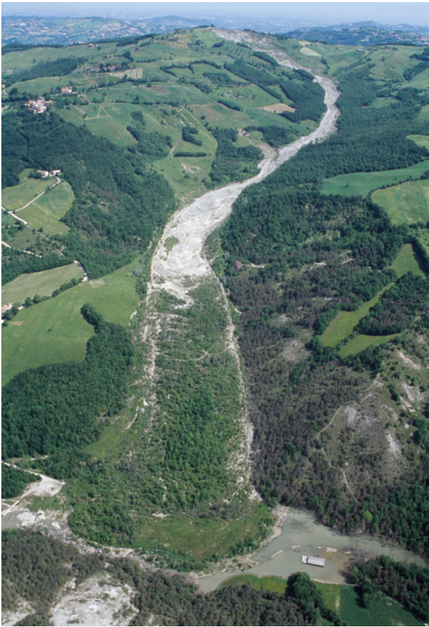
Fig. 18.7 The permanently active Roncovetro landslide (Reggio Emilia Province, photo G. Bertolini, 2012). The activity of the landslide is probably determined by the inflow of highly mineralized groundwater mixed with methane, coming from the subsurface (Bertolini 2010)
