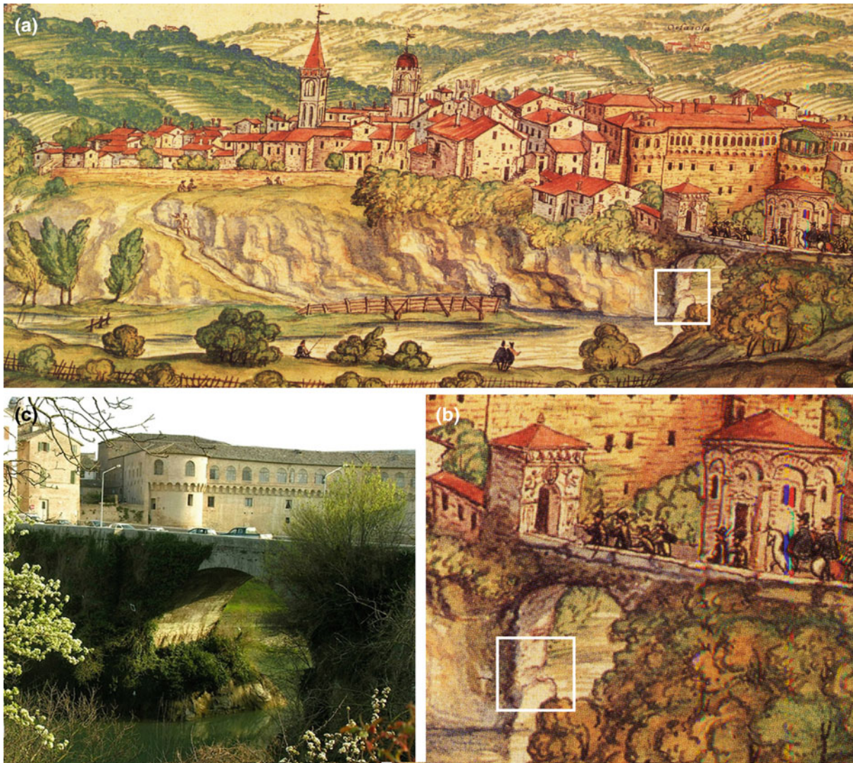
Fig. 22.5 The town of Urbania with the Riscatto Bridge in a drawing by Mingucci (1626) (a). In detail (b), the groove present in the bridge arches, indicative of the presence of a structure that closed the bridge, is
