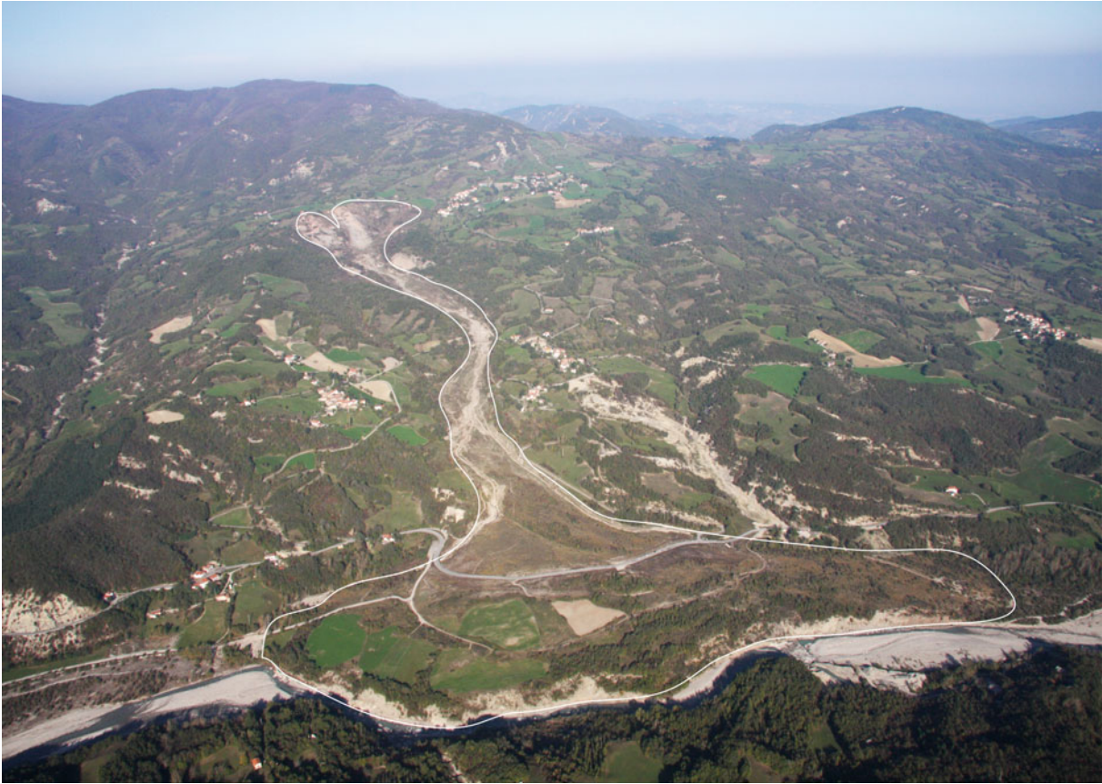
Fig. 18.9 The Signatico landslide, reactivated in 1977 (Parma Province, photo G. Bertolini, 2014). There were several previous reactivation events: ninth century, 1710, nineteenth century and 1906, causing formation of a dammed lake (Tellini and Chelli 2003)
