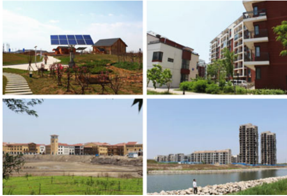
Fig. 3 On-site pictures of Tangshan Bay Eco-city in 2013 (Photos taken by Tian, Xinxin)
