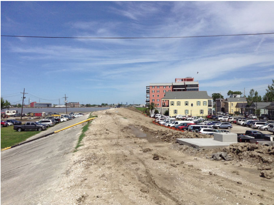
Fig. 1.3 Mississippi river levee at Algiers, Louisiana, directly opposite New Orleans Photo R. McLeman
