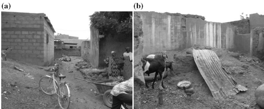
Fig. 4.4 Sloping street and destroyed houses in Kaya settlement. Photos by authors
