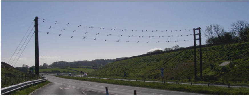
Fig. 3.5 The most common bat gantry design in the UK—steel wires with plastic spheres at intervals that are intended to be acoustic guides for bats
