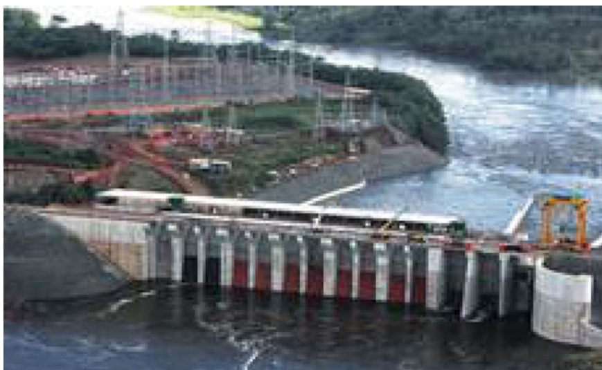
Fig. 2.13 Bujagali hydropower station on River Nile in Uganda
