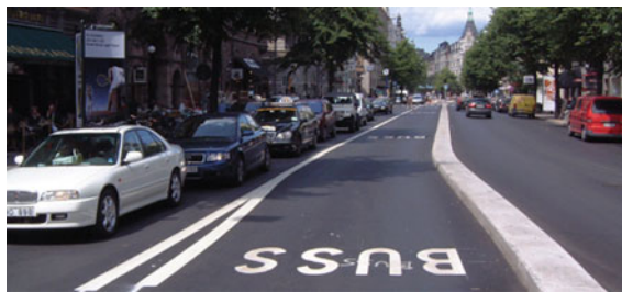
Fig. 2.12 Public transport reserved lanes in the middle in one direction at Sturegatan, Stockholm. This particular lane also serves as a “queue jumper” (photograph K Kottenhoff)
