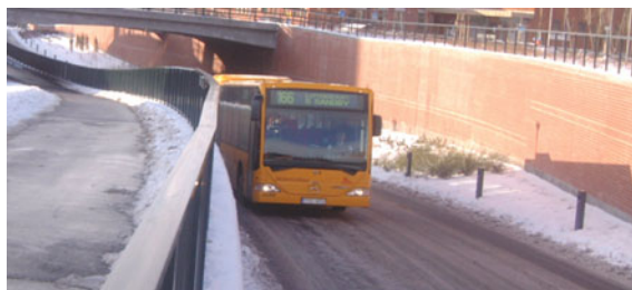
Fig. 2.11 Lundalänken in Lund, Sweden, is a partially separated “light busway”, here passing under an ordinary road. There is a parallel bikeway ( photograph K Kottenhoff)
