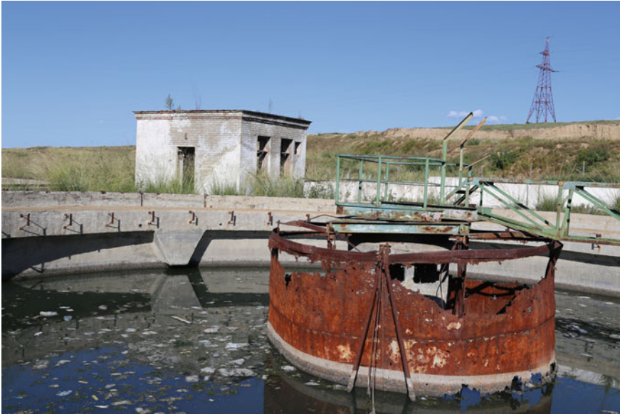
Fig. 25.6 Current state of Darkhan's central wastewater treatment plant
