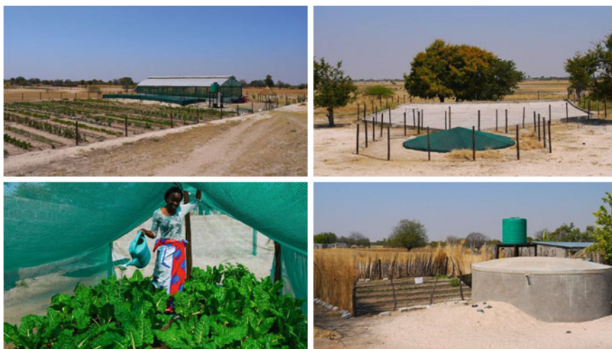
Fig. 26.7 Rainwater harvesting pilot plants (from top left clockwise : Green Village with greenhouse and outside garden, Green Village ground catchment with underground tank, household ferrocement tank with garden, spinach inside household greenhouse)
