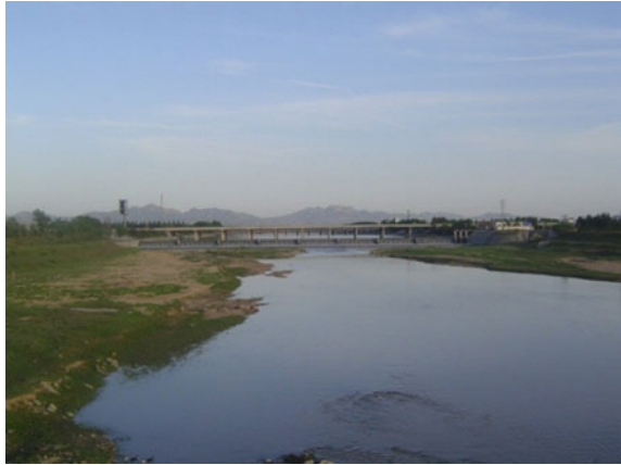
Fig. 24.2 Upriver view at the dammed Huangshui River
