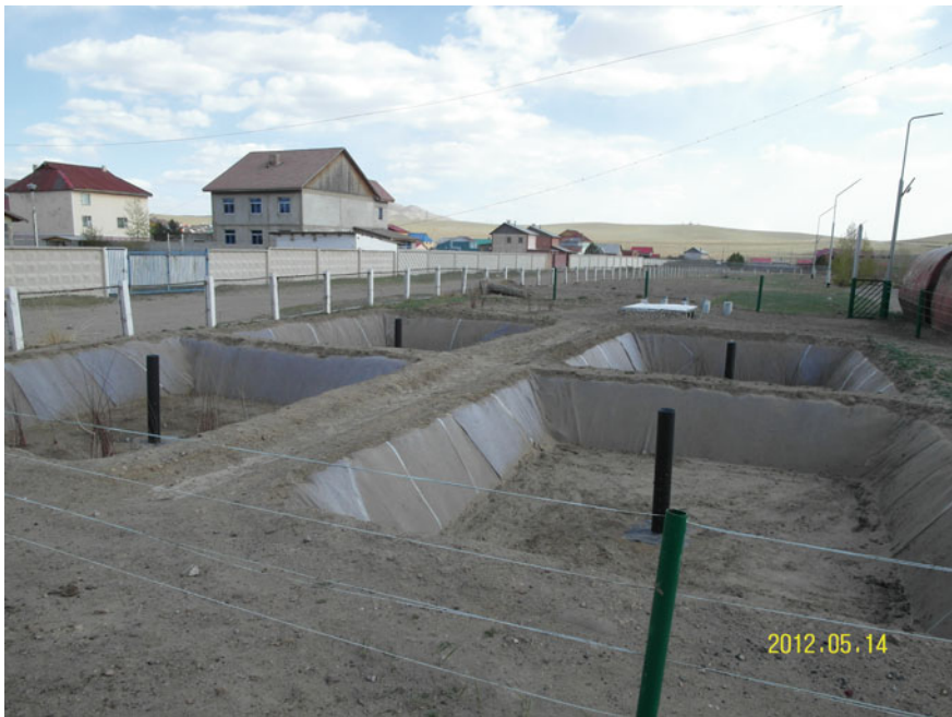
Fig. 25.11 Construction of the willow-based treatment beds
