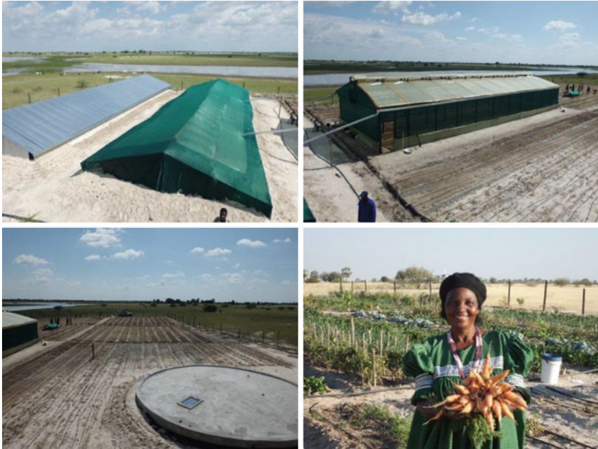
Fig. 26.8 Floodwater harvesting pilot plant (from top left clockwise : covered ponds, greenhouse, crops from outside gardens, underground tank and outside gardens)
