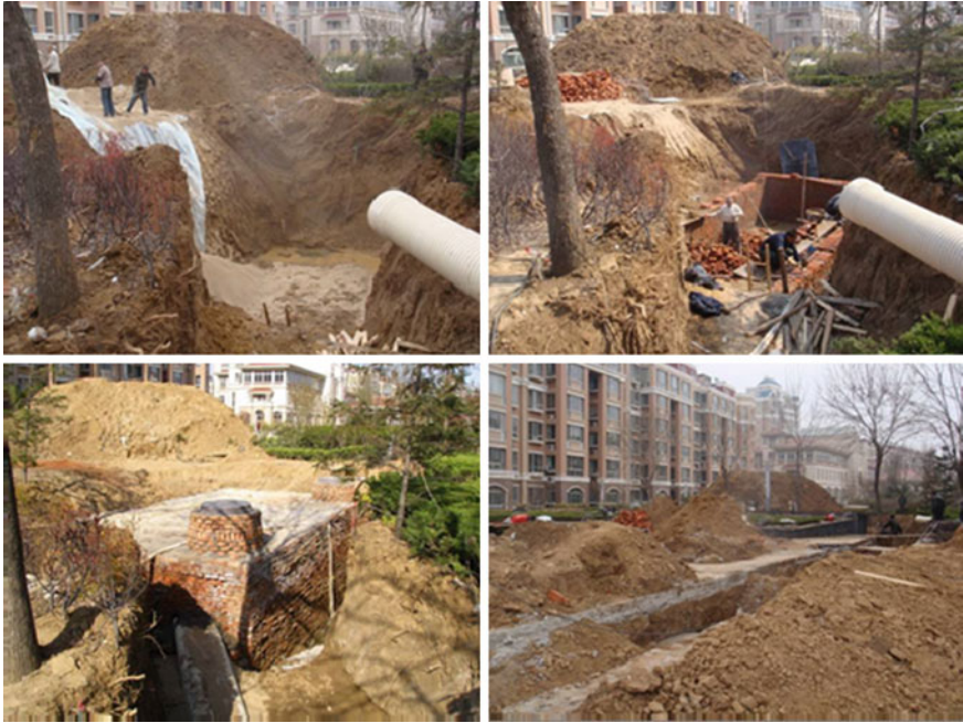
Fig. 24.11 Construction site of rainwater harvesting in Songfeng residential area
