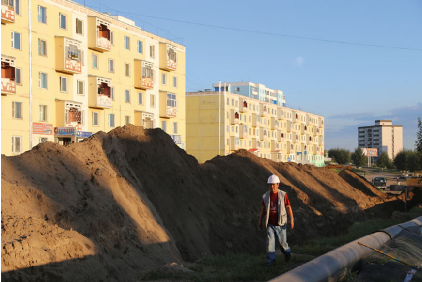
Fig. 25.5 Exchange of pipelines in Darkhan. Photo Daniel Karthe
