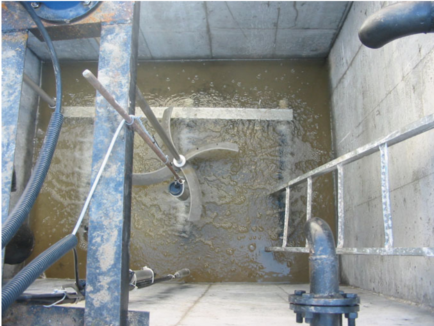
Fig. 25.8 View into the reactor while aeration testing in August 2011. At the bottom membrane tube aerators, above four-bladed stirrer, aside online sensors and inflow pipes. Photo Martin Vocks
