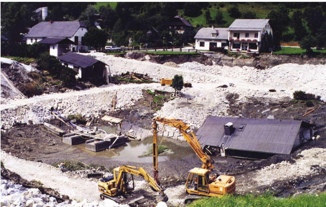
Fig. 10.12 An example of caving above mine workings (talc) intercepting saturated alluvium that then flowed into mine – the white material is silica rock used to stabilise inflow (After Galvin 1998)
