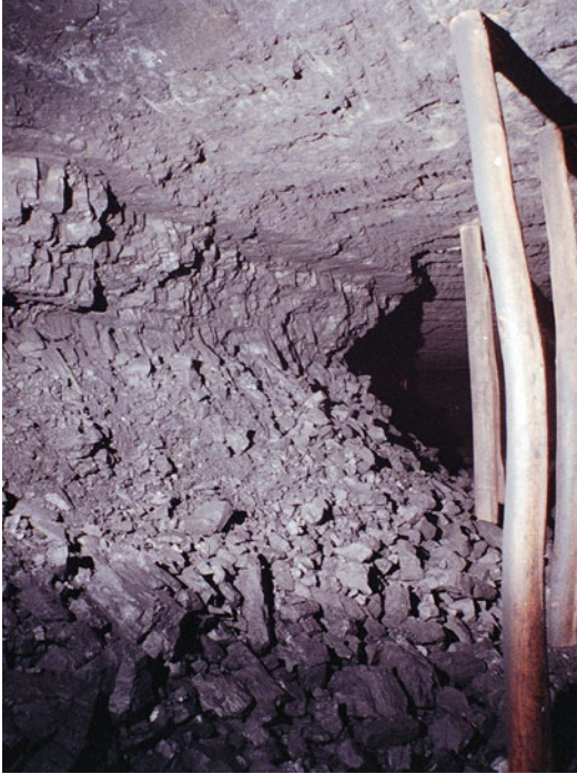
Fig. 4.13 A highly stressed pillar in high friction and cohesion contact conditions, resulting in the pillar taking on an hourglass shape
