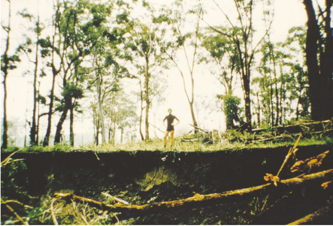
Fig. 11.10 An example of a pillar system failure that was bounded on one side by a geological fault
