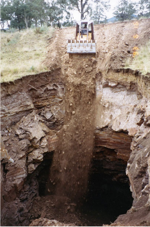
Fig. 3.34 Intersection failure over thick seam bord and pillar workings at shallow depth
