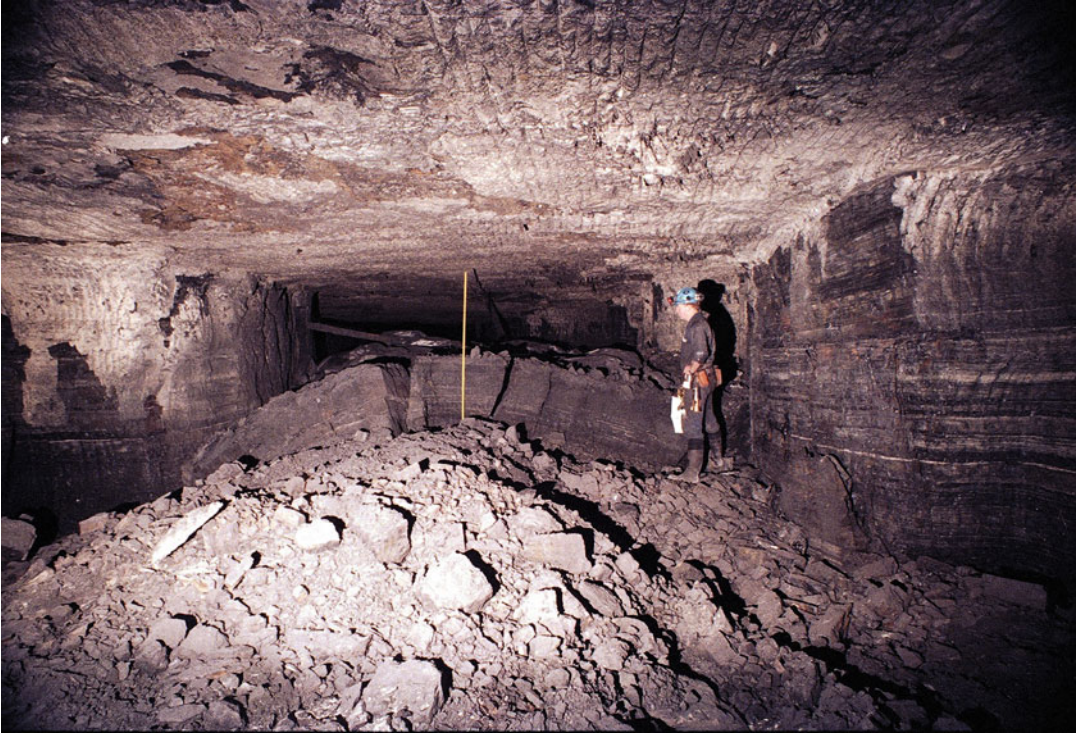
Fig. 4.35 Floor heave associated with the swelling of a claystone floor with a high montmorillonite content
