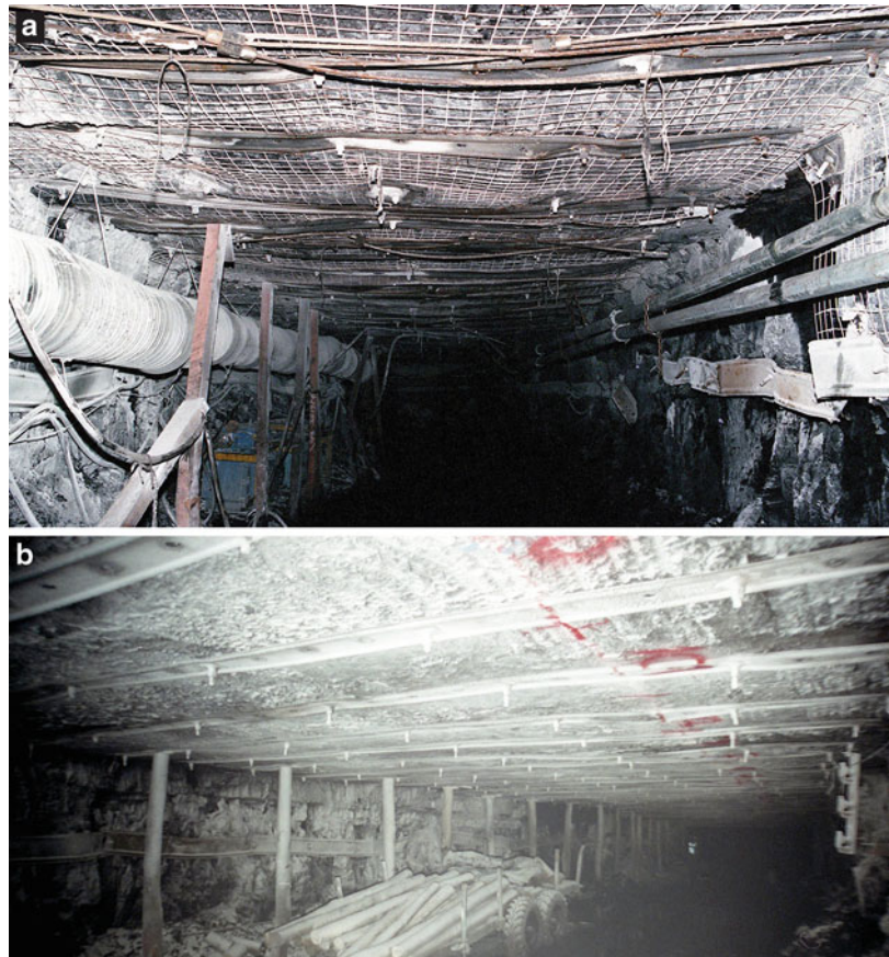
Fig. 9.24 An example of the beneficial effect on ground control of utilising a sacrificial roadway to create a lateral stress shadow in a high horizontal stress environment. (a) A 4.8 m wide cut-through driven at \sim 65^\circ to the regional major horizontal stress, which was \sigma_1 (b) An 8 m wide longwall installation roadway driven from the cut-through shown in (a) after the formation of a 10 m wide caved sacrificial roadway some 9 m further inbye
