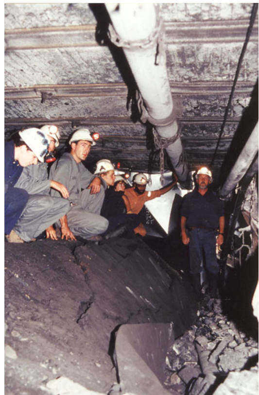
Fig. 9.7 Dynamic heave of a coal floor beam in a gateroad located adjacent to a highly loaded chain pillar
