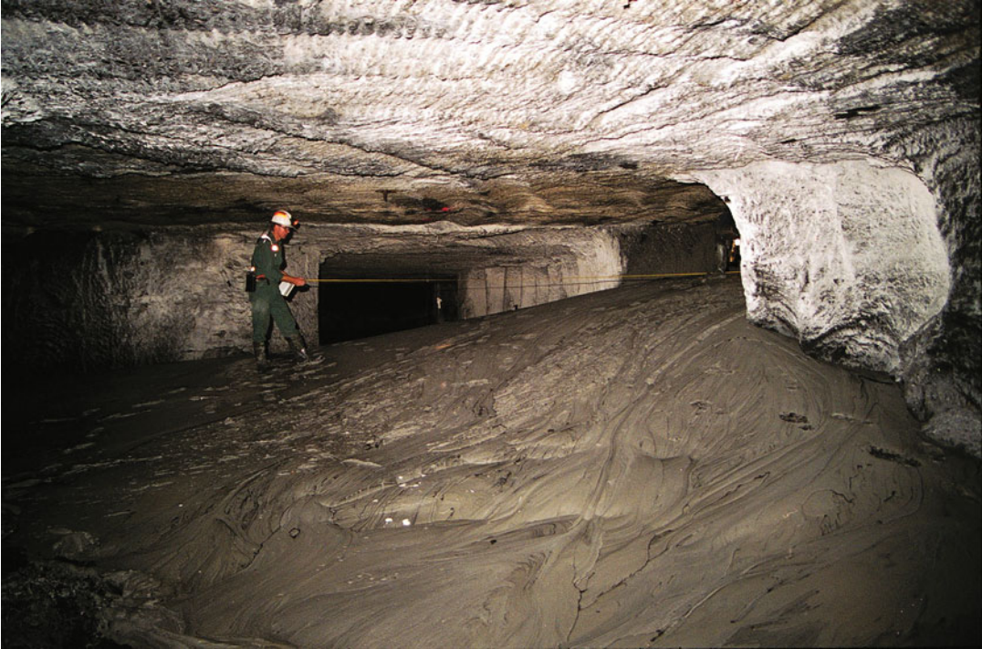
Fig. 11.11 Bord and pillar workings in the process of being backfilled with flyash paste, Awaba Colliery, Australia
