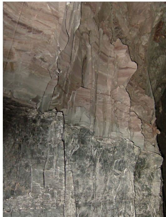
Fig. 11.13 A fall of roof material which has a similar rock mass strength to the coal seam, thereby resulting in an increase in the effective height of the pillar
