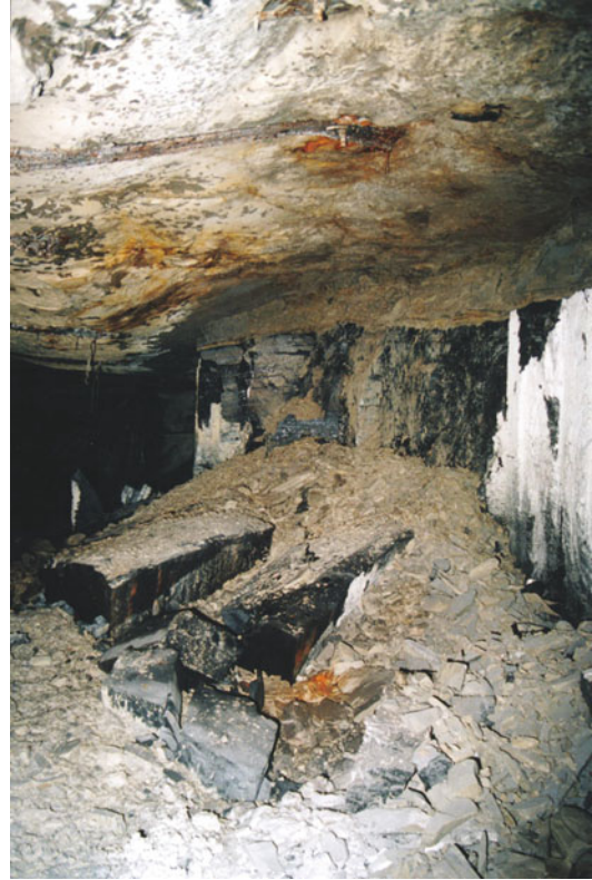
Fig. 4.14 Blocky rib spall along cleat planes due to induced lateral tension caused by extrusion at the pillar/roof interface of a claystone with low cohesive and frictional properties
