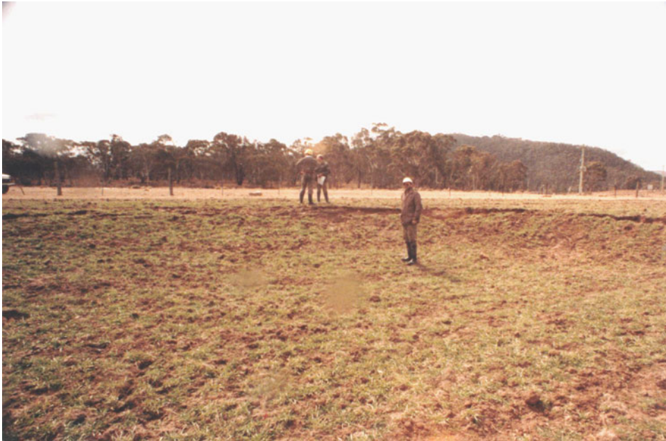
Fig. 3.36 Surface expression of a sudden overburden failure event associated with pillar extraction panel at shallow depth
