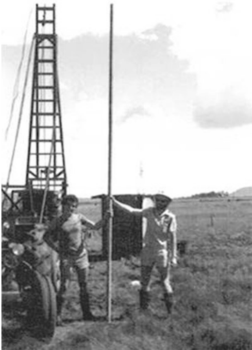
Fig. 3.23 A length of core recovered from a dolerite sill illustrating the lack of bedding planes in the material and its high intact strength (After Galvin 1981)
