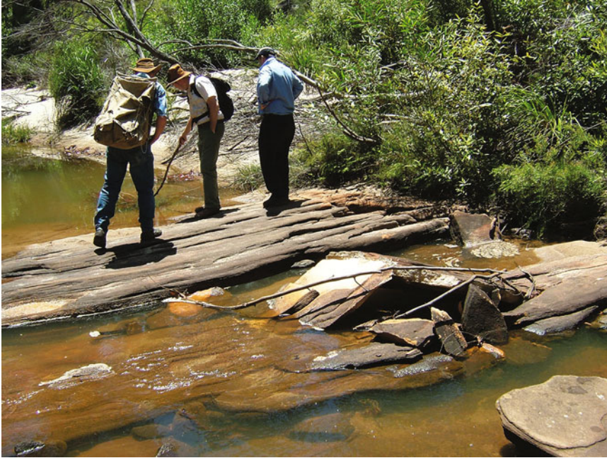
Fig. 10.30 Buckling of near surface strata in a watercourse subjected to upsidence and valley closure
