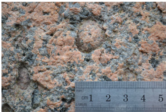
Fig. 1 Surface roughening of the granite rapakivi (St. Petersburg, Facade of Russian museum building)
