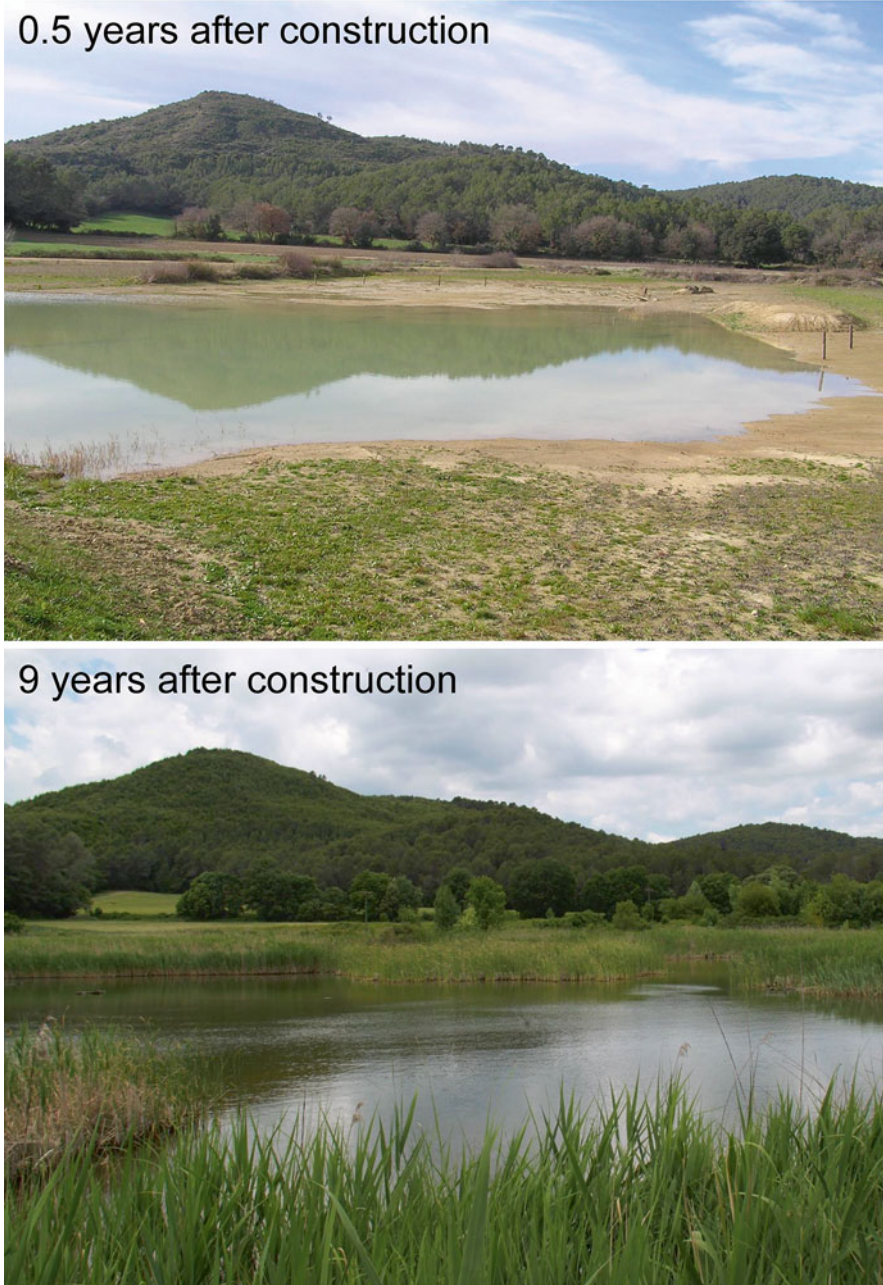
Fig. 15.7 CW for biodiversity enhancement close to Banyoles, Catalonia. The goal of this CW was to increase amphibian populations within the framework of the LIFE-Nature project LIFE03 NAT/E/000067. The upper picture shows bare shores and scarcity of macrophytes 0.5 years after wetland construction; the lower picture shows the dense macrophyte community (dominated by common reed Phragmites australis and cattail Typha latifolia ) that established shortly after (still present)
