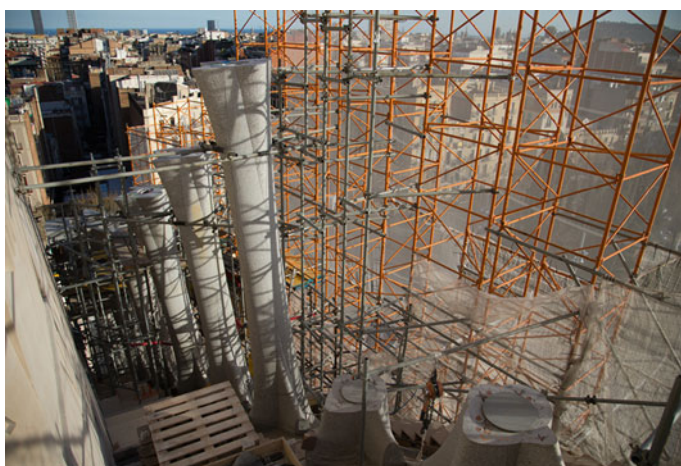
Fig. 24 Narthex colonnade under construction (2014)
