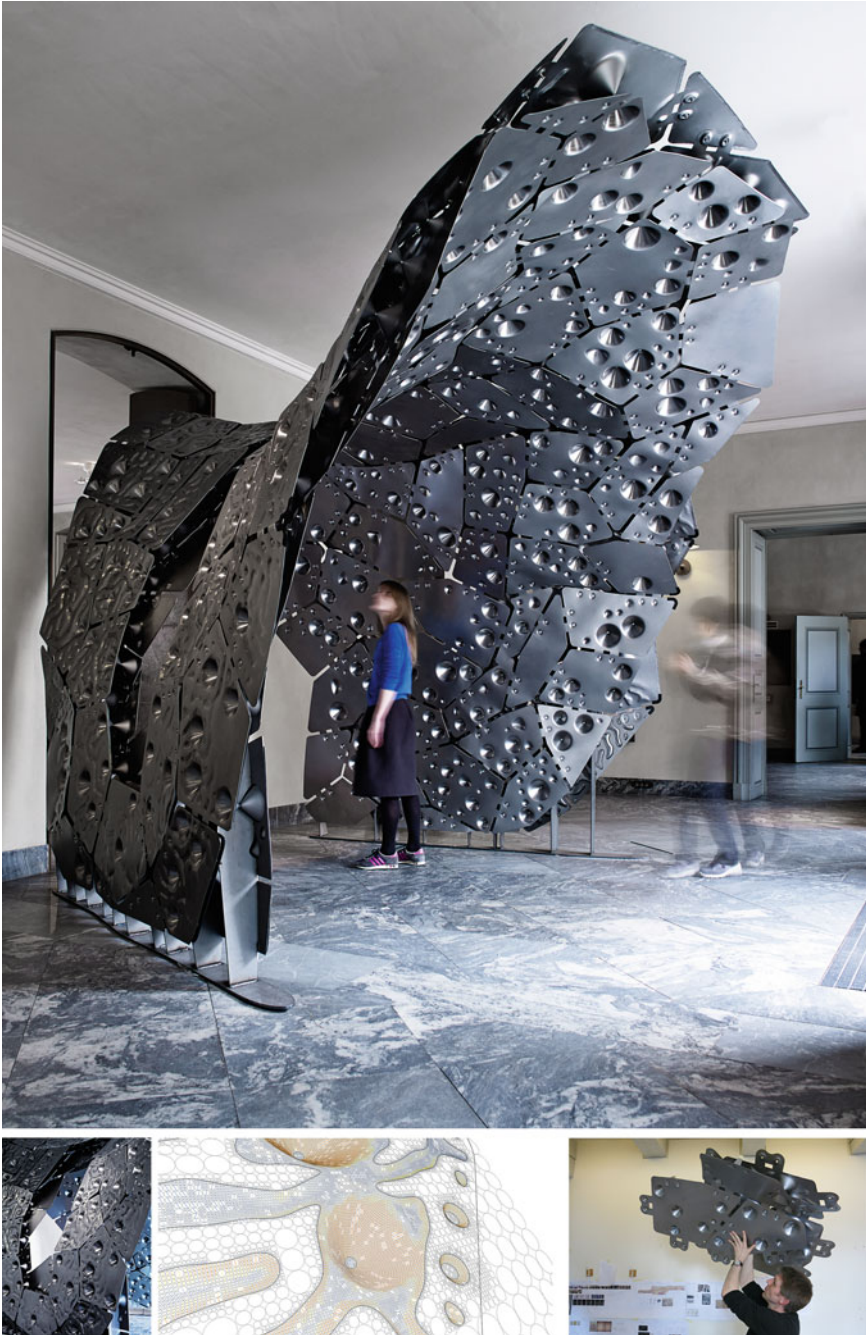
Fig. 9 Stressed Skin is a dual skin in which deep incrementally pressed indentations form the connections between the skins and further corrugation achieves stiffness
