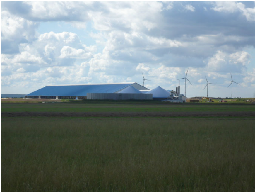
Fig. 1 Example of a stable system for milk production with biogas plant for the production of electricity and heat (location near Frankfurt an der Oder, Germany). Surrounding lands and water bodies are subject to increased risk of nutrient pollution. Land management requires mandatory high standards for the protection of water resources
