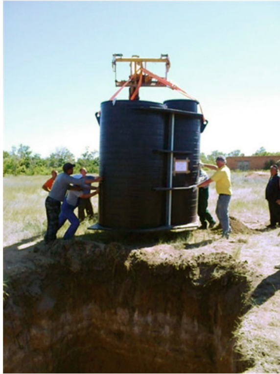
Fig. 1 Installation of the PE-HD lysimeter station at the Poluyamki test farm (photo E. Stephan)
