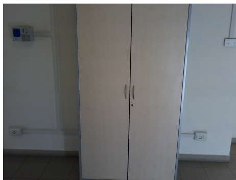
Fig. 6: Setting in which the command “go to the socket near the closet” has an ambiguous meaning. The command, in fact, could be grounded with either the socket on the left or the one on the right of the image, since they are both near the closet.
