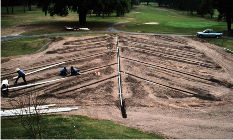
Fig. 2.30 A herringbone drainage pattern is commonly used for golf green and sports fields
