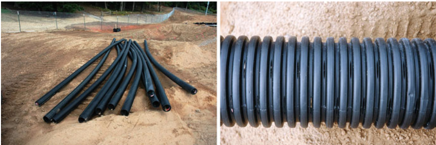
Fig. 2.19 Corrugated tile pipe is widely used for golf course drainage ( left ). A smooth inner-walled pipe should be considered for increased drainage efficiency. Slits in pipes where water enters ( right )
