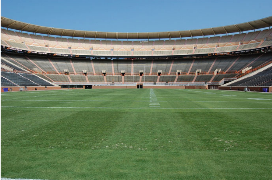
Fig. 2.7 Surface slopes are generally between 1 and 3%. This greatly enhances surface water drainage without compromising play
