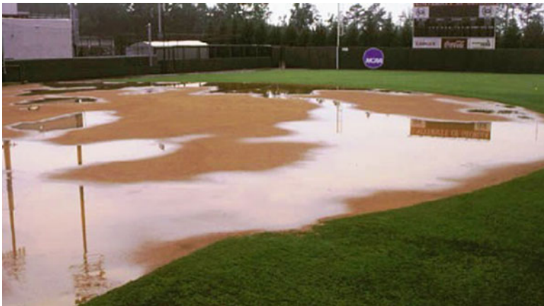
Fig. 2.53 Surface drainage is necessary for highly compacted, clay content surfaces such as softball and baseball infields
