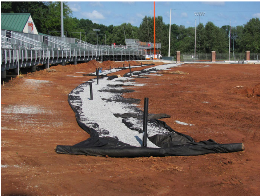
Fig. 2.55 Installing a perimeter drainage line adjacent to the warning track of a baseball field
