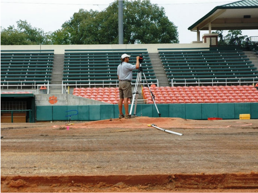
Fig. 2.28 Checking the integrity of settled drain lines to ensure continuous fall to facilitate proper drainage
