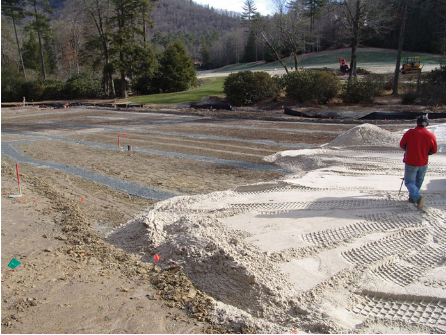
Fig. 2.39 Sand capping a perpetually wet site to raise the turf above the naturally occurring high water table
