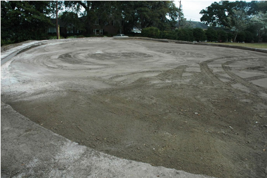
Fig. 2.27 Subgrade of golf greens should be within 1 in (2.5 cm) of the eventual surface grade to facilitate more even drainage and soil moisture. Otherwise, shallow soils tend to stay saturated while deeper soil remain excessively dry
