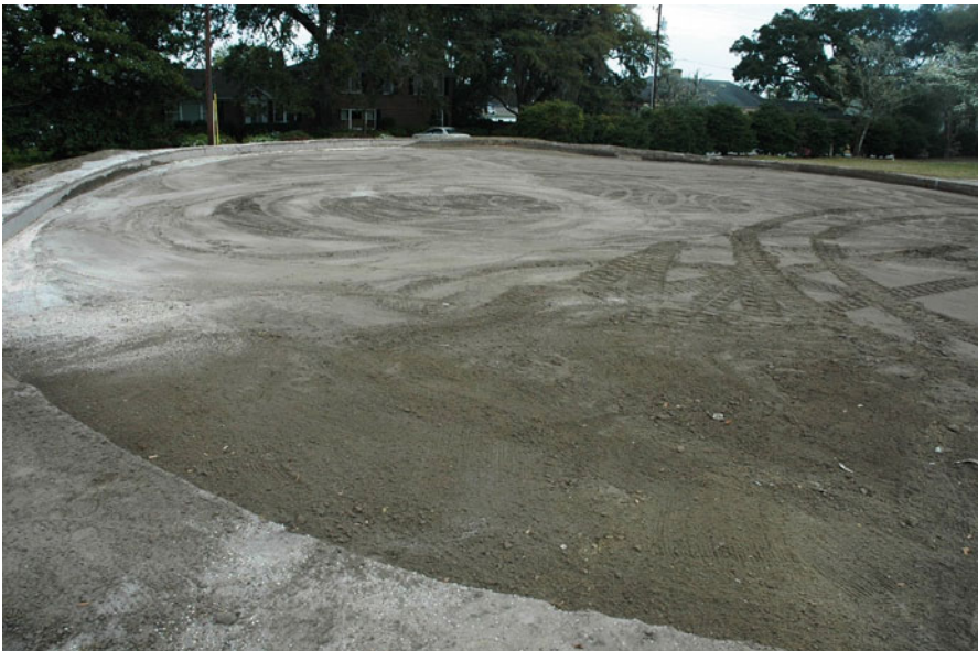
Fig. 2.27 Subgrade of golf greens should be within 1 in (2.5 cm) of the eventual surface grade to facilitate more even drainage and soil moisture. Otherwise, shallow soils tend to stay saturated while deeper soil remain excessively dry
