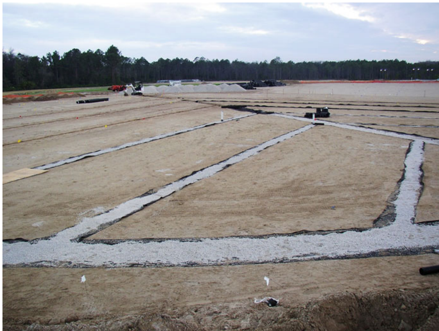
Fig. 2.56 More extravagant drainage systems along with a sand-based rootzone commonly used on collegiate and professional baseball fields
