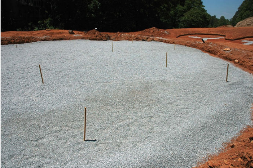
Fig. 2.32 Grade stakes to clearly mark proper depths of various components of layered systems
