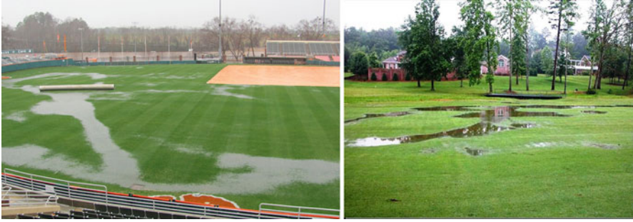
Fig. 2.1 Improper or inadequate drainage is a very common agronomic problem cited by sports field managers ( left ) and golf course superintendents ( right )
