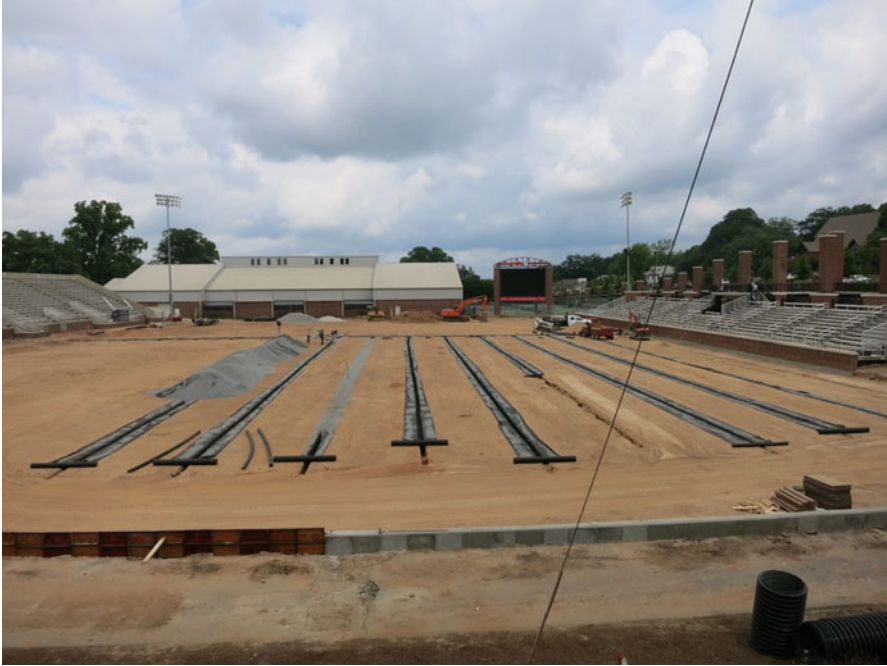
Fig. 2.43 A sand-based sports field with drainage lines imbedded into the subgrade to facilitate subsurface water removal
