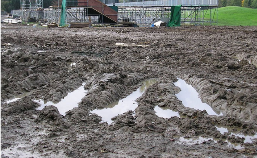
Fig. 2.6 Excessive soil moisture acts like a lubricate allowing soils to be damaged when saturated and exposed to uncontrolled traffic
