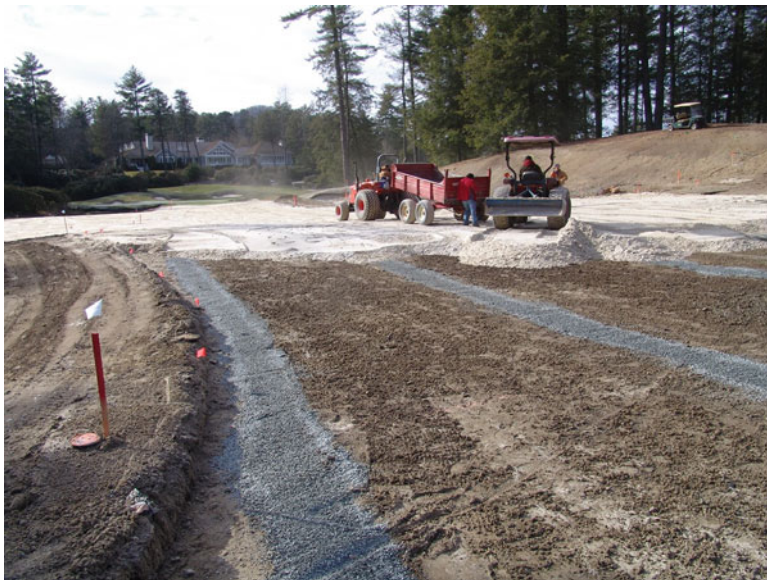
Fig. 3.26 Sand capping a golf course fairway can provide desired results if appropriate soil science is used in determining needed sand depth and drain tile spacing
