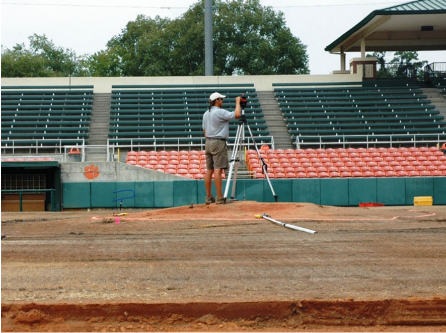
Fig. 2.28 Checking the integrity of settled drain lines to ensure continuous fall to facilitate proper drainage
