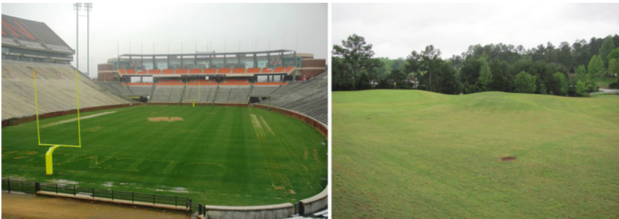
Fig. 2.2 A combination of surface and subsurface drainage systems are needed for high profile turf venues which must play regardless of weather conditions. Left illustrates a “crowned” sports field with sideline drains which capture surface runoff while right demonstrates surface contouring to redirect excessive surface runoff away from a golf green
