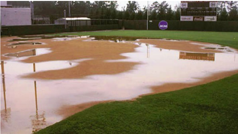
Fig. 2.53 Surface drainage is necessary for highly compacted, clay content surfaces such as softball and baseball infields
