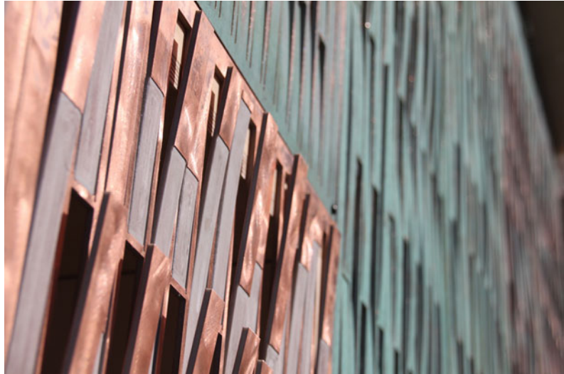
Fig. 9 Detail of behavioural composites created through the organisations of expanding and contracting composite layers
