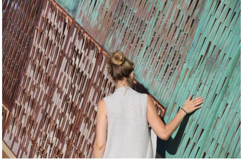
Fig. 5 Full scale three-by-eight-meter prototype, including 24 composite behavioural panels and the embedded sensor network for post construct analysis
