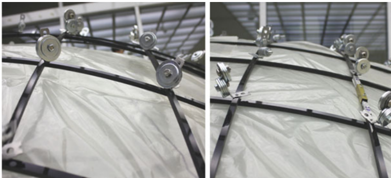
Fig. 9 Separation between pneumatic falsework and grid due to gradual deflation in end state ( left ). Re-established contact between cushion and grid after re-inflation ( right ).
