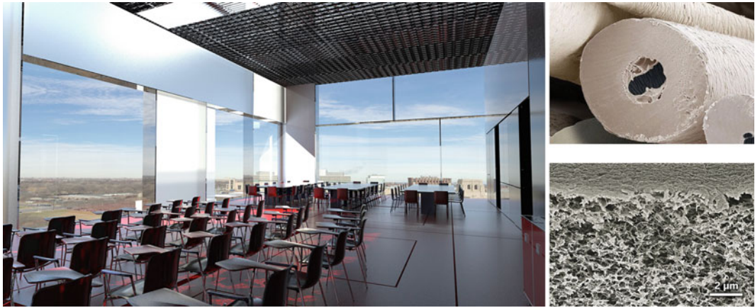
Fig. 12 Left Biomimetic design through advanced materials, as a polar bear's coat is clear yet appears white so does the skin of the building allowing for passive solar
