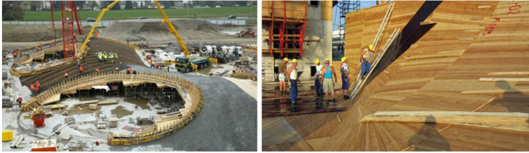
Fig. 1 Formwork for concrete structures ( Image B+G, design to production )
