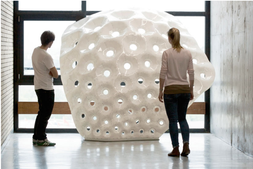
Fig. 13 The full-scale mock-up was built of PET-G plates with a thickness of only 0.5 and 0.75 mm
