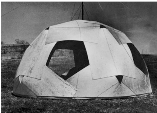
Fig. 1 Two-frequency geodesic pldome in Des Moines, Iowa, 1957. The hemisphere spans 7.3 m and is made out of marine plywood sheets with a thickness of 6.4 mm. (Marks 1973, p. 210)
