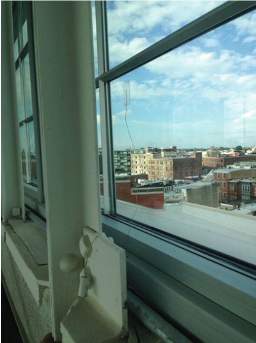
Fig. 9 Installed glazing surface temperature sensor
