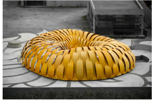
Fig. 2 ICD/ITKE research pavilion 2010 spans 10 m and consists of 80 birch plywood strips with a thickness of 6.4 mm
