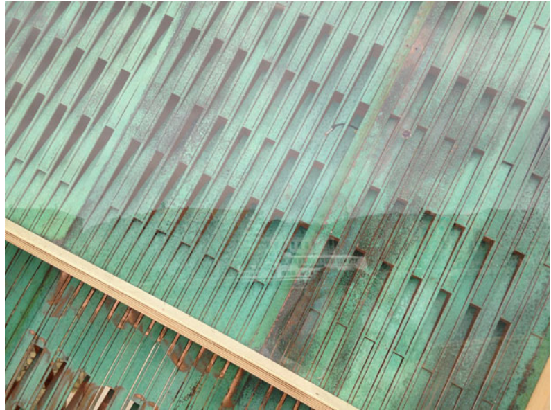
Fig. 6 A case with transparent acrylic plate installed on the external side of the membrane. It is possible to see the thermal and light sensors installed between the acrylic plate and the membrane just above and to the right of the image centre. Viewing the membrane through a transparent plate also modifies the visual appearance, as reflections of the context become visible
