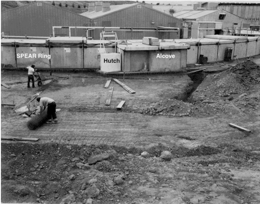
Fig. 3.4 Picture of the SPEAR accelerator housing modified by rearranging shielding blocks to add an alcove that housed the exit port and monochromator shown in Fig. 3.2. The white box attached to the outside of the accelerator housing is the X-ray hutch that housed the sample chamber and, as shown in the picture, was located outdoors and covered by a plastic sheet when it rained. In parallel with the Pilot Project photoemission experiments, construction was taking place to build the first SSRL experimental hall
