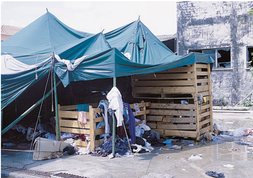
Fig. 2.4 Temporary shelter, Turkey earthquake (1999)
