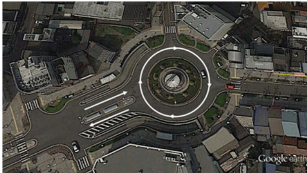
Fig. 1 Roundabout intersection at Ichinomiya
