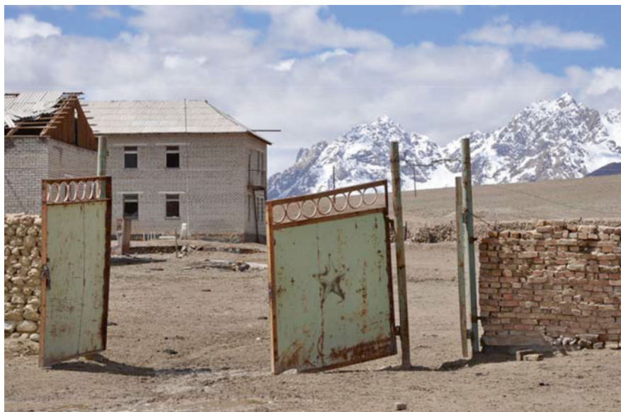
Fig. 3 Anandoned border post ‘Ozernaja’ of the Russian Border Forces (RBF), Tokhtamysh area of the Eastern Pamirs. After the pulling-back of the RBF, funds for the Tajik border forces were insufficient to maintain existing border infrastructure (Photograph © T. Kraudzun, Jun 2010)
