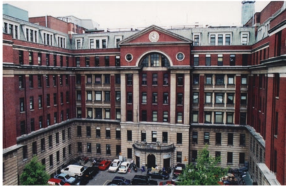
Fig. 1 The Middlesex Hospital, London, UK (founded 1745; 2005, replaced by the new University College London Hospital). Image courtesy of University College London Hospital NHS Trust archive
