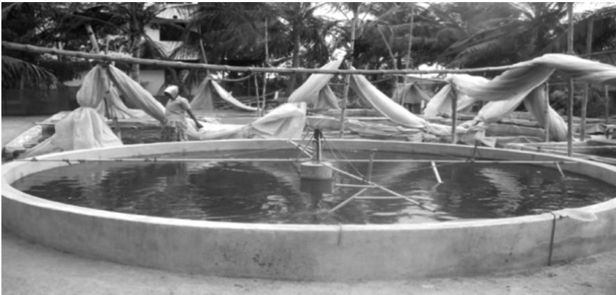
Fig. 7.4 Circular concrete tank of 3 m radius.
