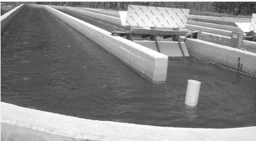
Fig. 2.2 Raceway pond for the large scale microalgae cultivation (200 m 3 ) at HighTech Algae Center, Hadong, South Korea.
