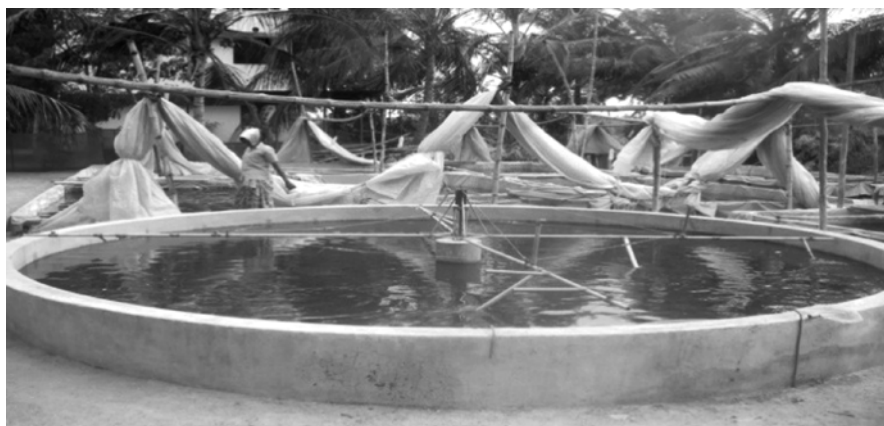
Fig. 7.4 Circular concrete tank of 3 m radius.
