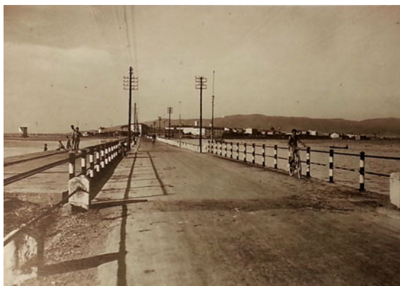
Fig. 3 The embankment and railway line, original postcard photograph, property of Dalle Nogare, Armetti and C., Milano (1939). In Savoi and Andruccetti (1994)
