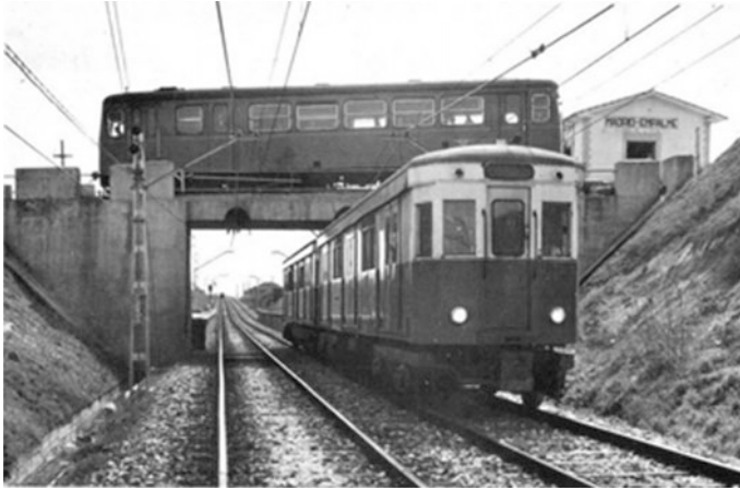
Fig. 4 Crossing between suburbano ( downstairs ) and almorox ( upstairs )
