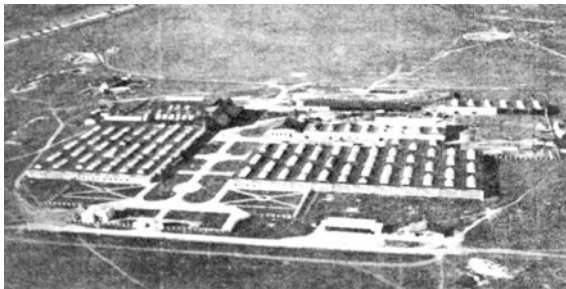
Fig. 7 Aerial view in 1929 (Salcă 2006)
