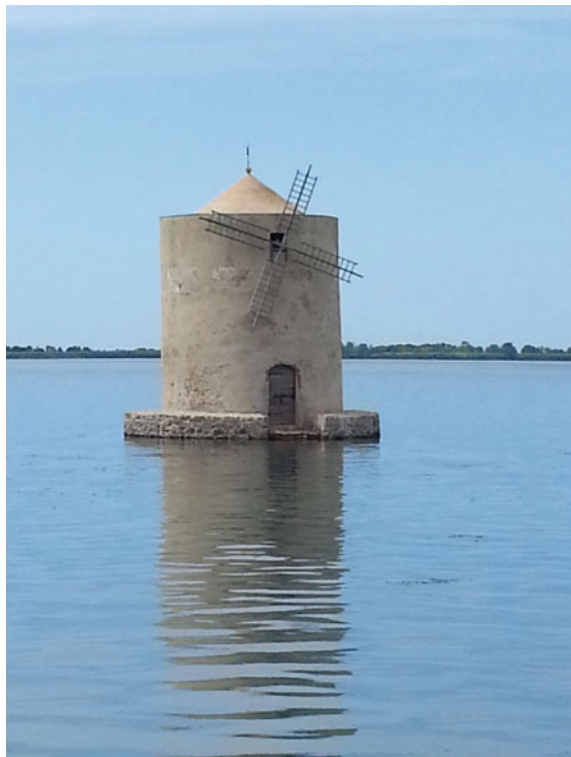
Fig. 10 Photograph of the mill today on the Orbetello Lagoon (Chiavoni 2012)
