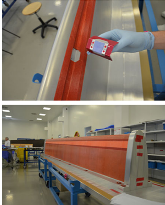
Fig. 12 Positioning of brackets and sparing out of the bracket heads with special cutting stamps ( top ); first skin layer applied on full span ( bottom ) (INVENT)
