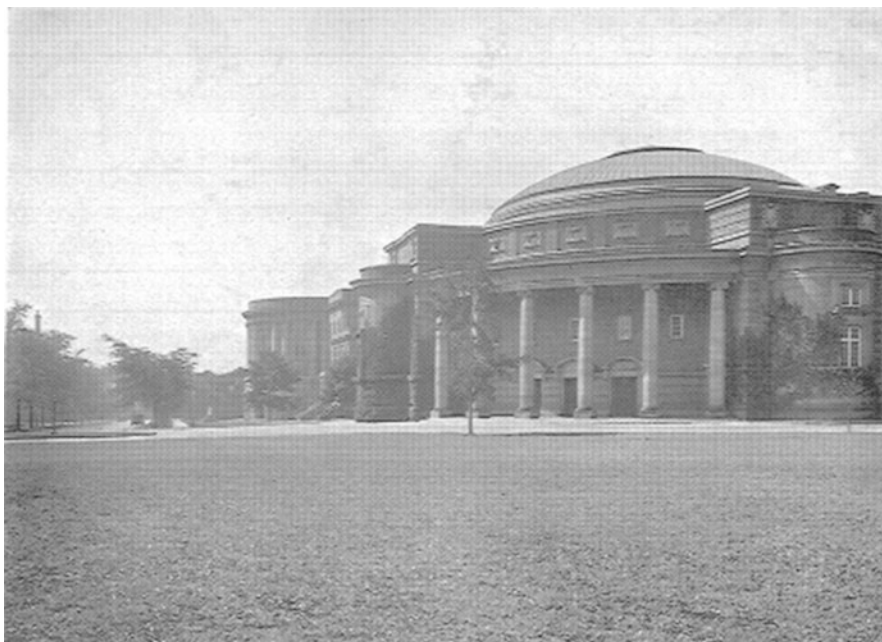
Fig. 3 Convocation Hall. Image from Fields (1928b) and reprinted with permission of the University of Toronto Press
