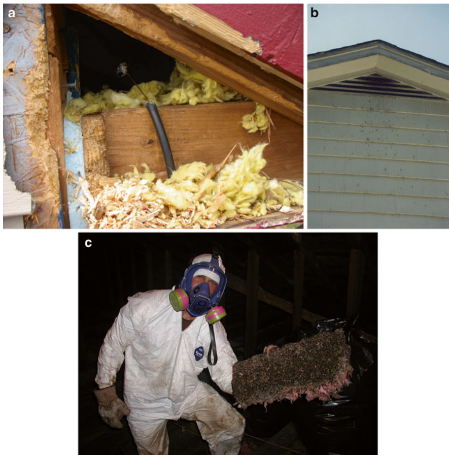
Fig. 9.5 (a) Framing, insulation, and wire damaged by a gray squirrel ( Sciurus carolinensis ). Photo by Kevin Cornwell. (b) Bat droppings staining the outside of this house. Photo by Stephen M. Vantassel. (c) Bat droppings covered this pink insulation enough to turn it black. Photo by Jason Reger
