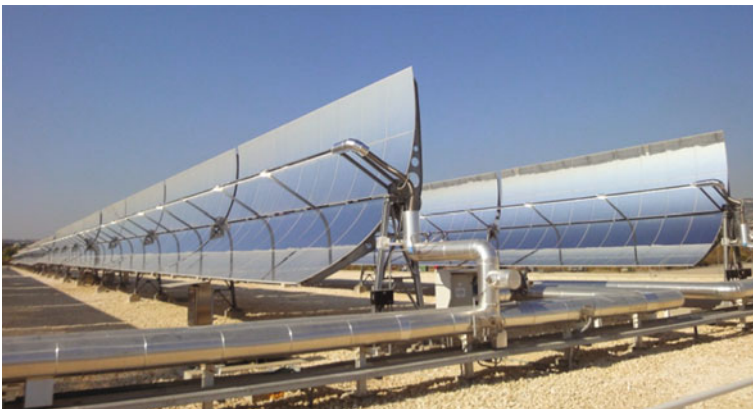
Fig. 2 String of solar collectors (Archimede 5 MW plant located in Priolo Gargallo, Sicily)
