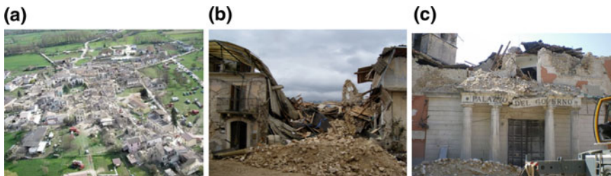
Fig. 3 Onna city after the April 6, 2009 seismic event struck (a, b); L'Aquila city (c)
