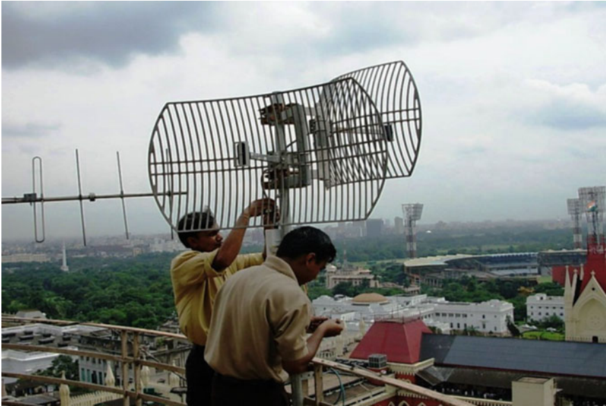
Fig. 10 Typical line of site alignment of SCADA radios
