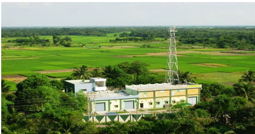
Fig. 9 Typical installation of radio base station at Naksa, N24 Pgs
