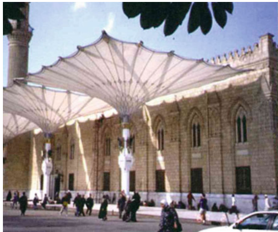
Fig. 3.7 A case of a seasonal structure designed for the summer, which offers shade and shelter from heat radiation, El Cairo, Egypt (Source Zanelli 2007)
